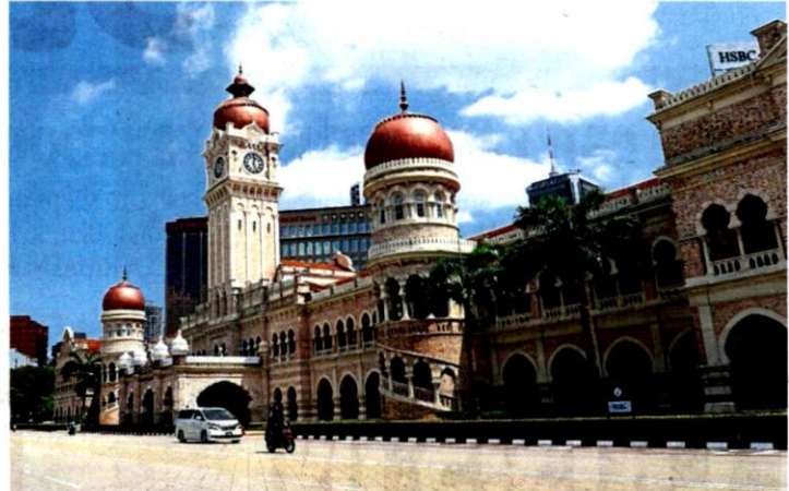
Iconic landmark: A general view of the Sultan Abdul Samad Building in the heart of Kuala Lumpur.
